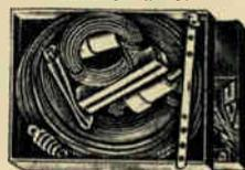
Complete in every detail and containing only the finest components, they will provide the ultimate in reception. This kit includes: 50 ft. 7/24 aerial wire, 50 ft. No. 20 insulated lead-in, 25 ft. ground wire, approved arrester, ground clamp, lead-in strip, two porcelain insulators, two nail-it knobs. Can be used with all types of broadcast and all-wave receivers.
